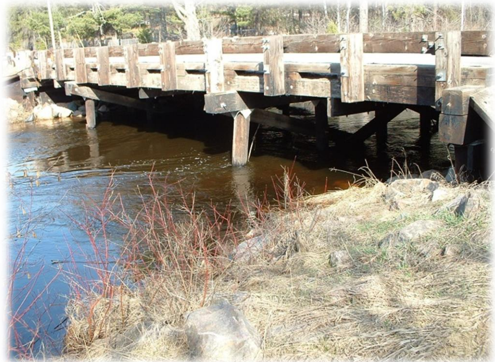
FIGURE 22 EAST BRANCH OF ESCANABA RIVER, FORSYTH TOWNSHIP
