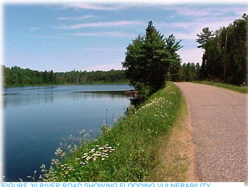
FIGURE 30 RIVER ROAD SHOWING FLOODING VULNERABILITY
