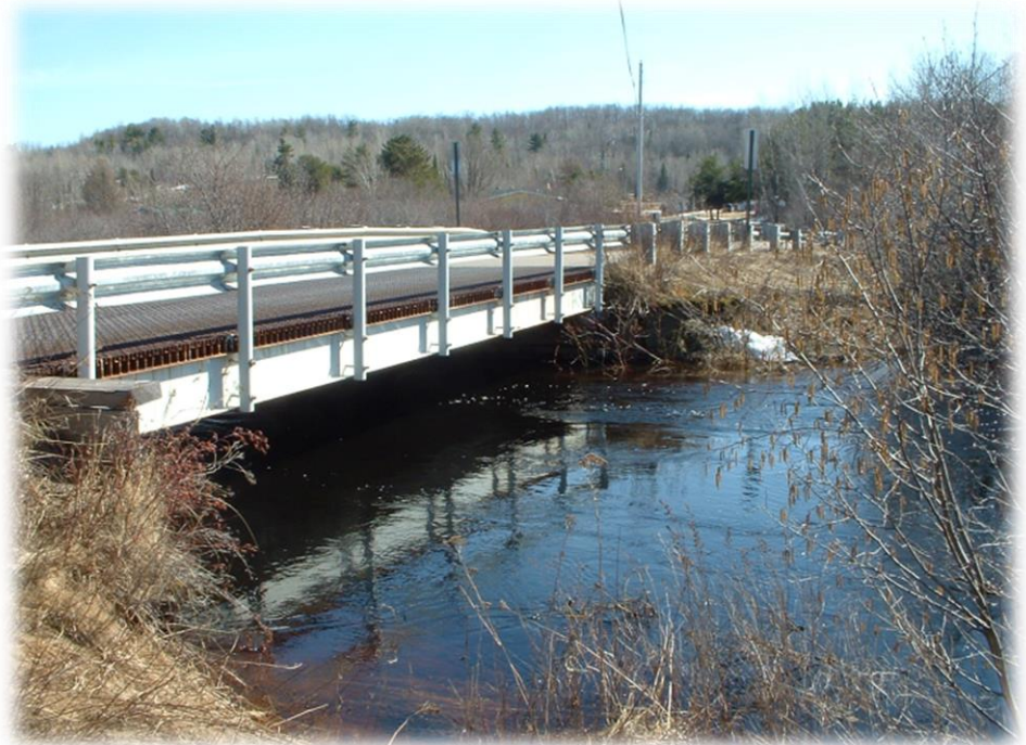
FIGURE 23 WOLF LAKE ROAD BRIDGE
