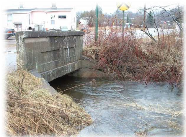
FIGURE 32 COUNTY RD PCC BRIDGE OVER ELY CREEK
