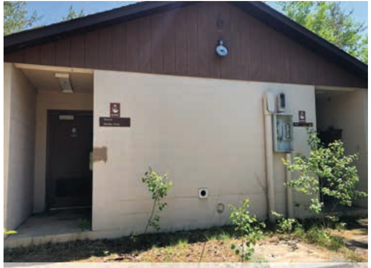
ABANDONED BUILDING ONE OF THREE ABANDONED BUILDINGS TO BE DEMOLISHED.
