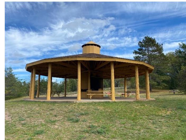
EXISTING LAKE TOP PAVILION
